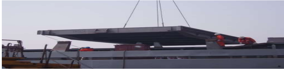
Fig 1.4: Lift-away hatch covers
