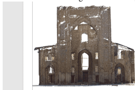
Fig. 7. The Facade of the Mausoleum Ishratkhana. Point cloud captured by Faro Focus 3D S120 laser scanner.
